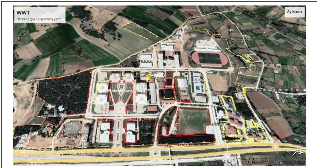
Wastewater treatment plant location
